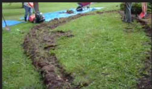
Build the berm with sod
