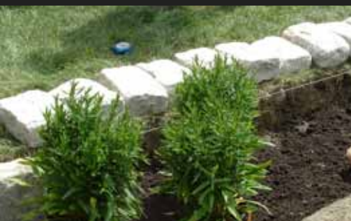
Create a berm with landscaping stone
